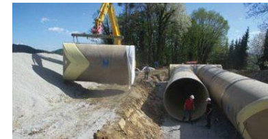
Water Pipeline Repair & Replacement
